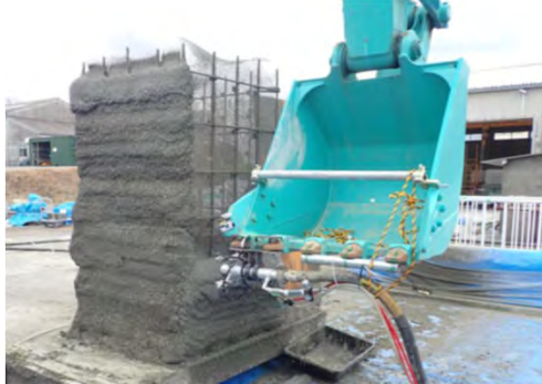
Shotcrete Printing 材料噴射
